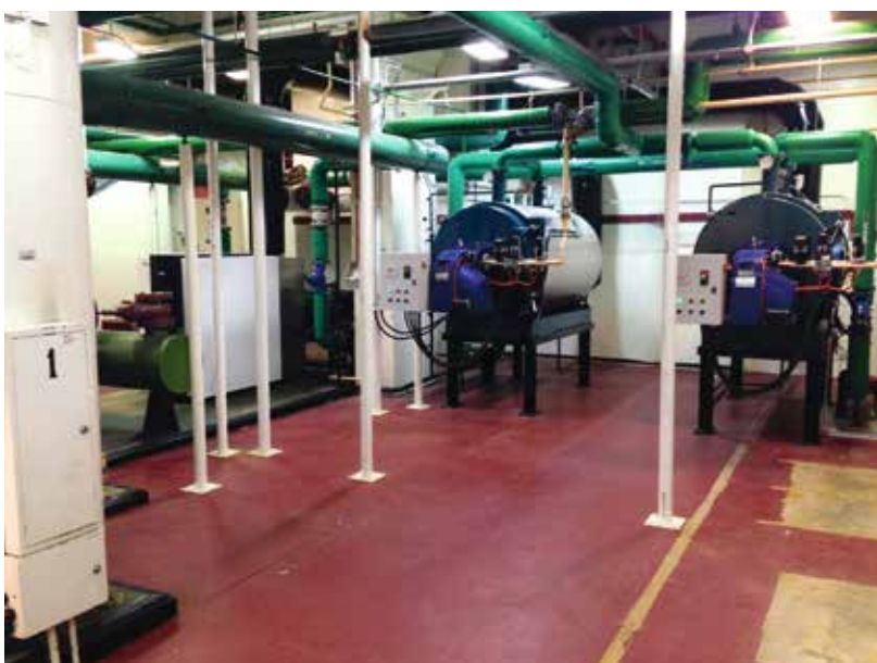
Boiler upgrade showing newly installed boilers in 2014. Photo: Kopievsky, M.AIRAH, Museum of Australian Democracy collection.
