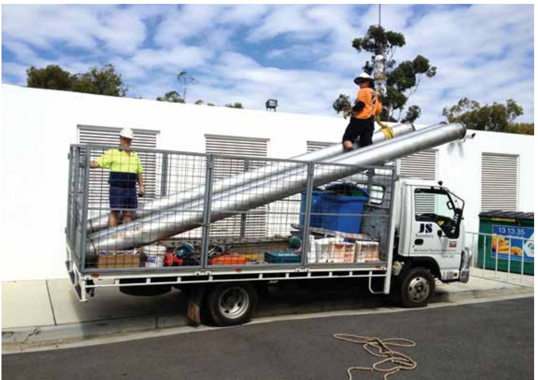
Installing the new chimney flues. Photo: J. Sainsbury
